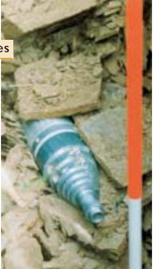
The GRUNDORAM for installing steel pipes up to DN 4000 and the GRUNDOMAT soil displacement hammer for house connections and crossings.
