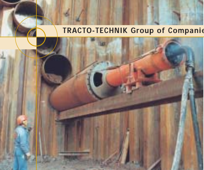
The GRUNDORAM for installing steel pipes up to DN 4000 and the GRUNDOMAT soil displacement hammer for house connections and crossings.
